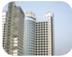
WanJie Hospital, China
